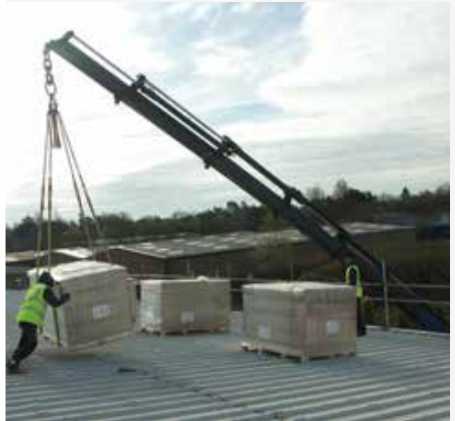
Solar panels being lifted onto the roof.
