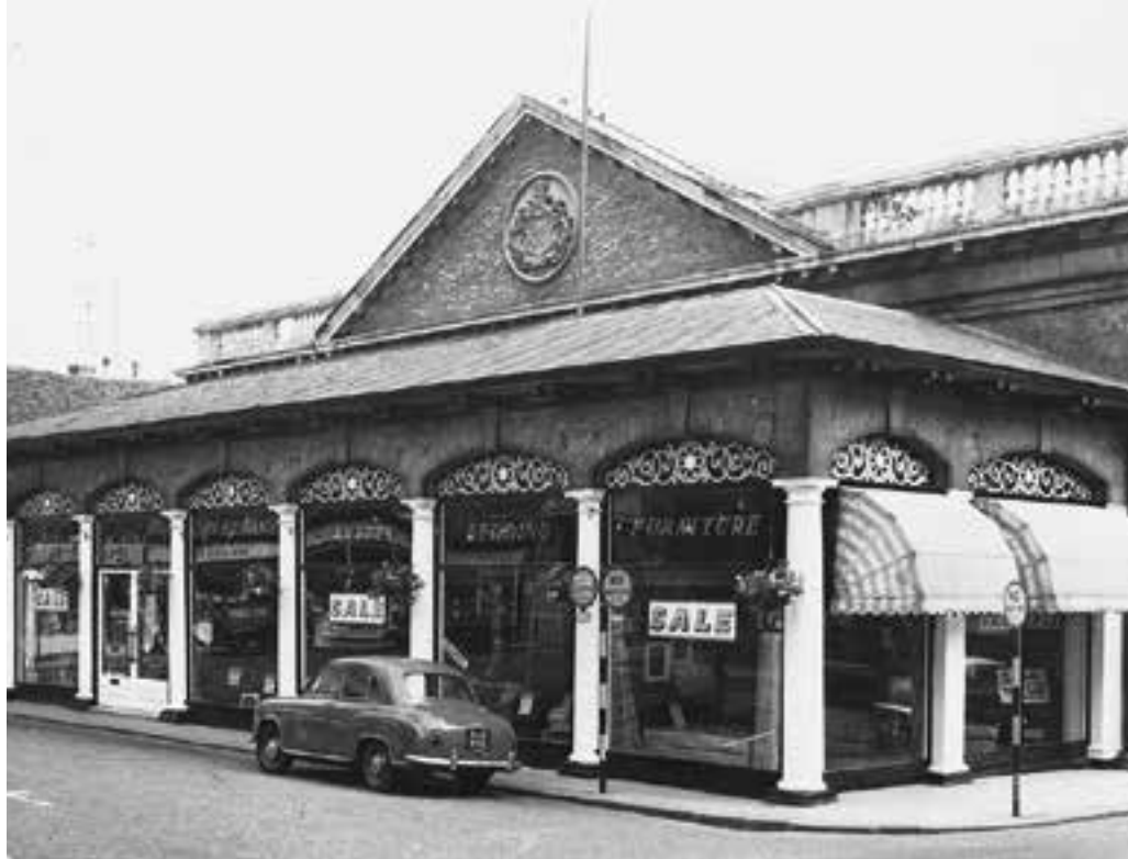
The Corn Exchange showroom in Bury St Edmunds. When Glasswells took it over it was one of the biggest display windows in the region.
