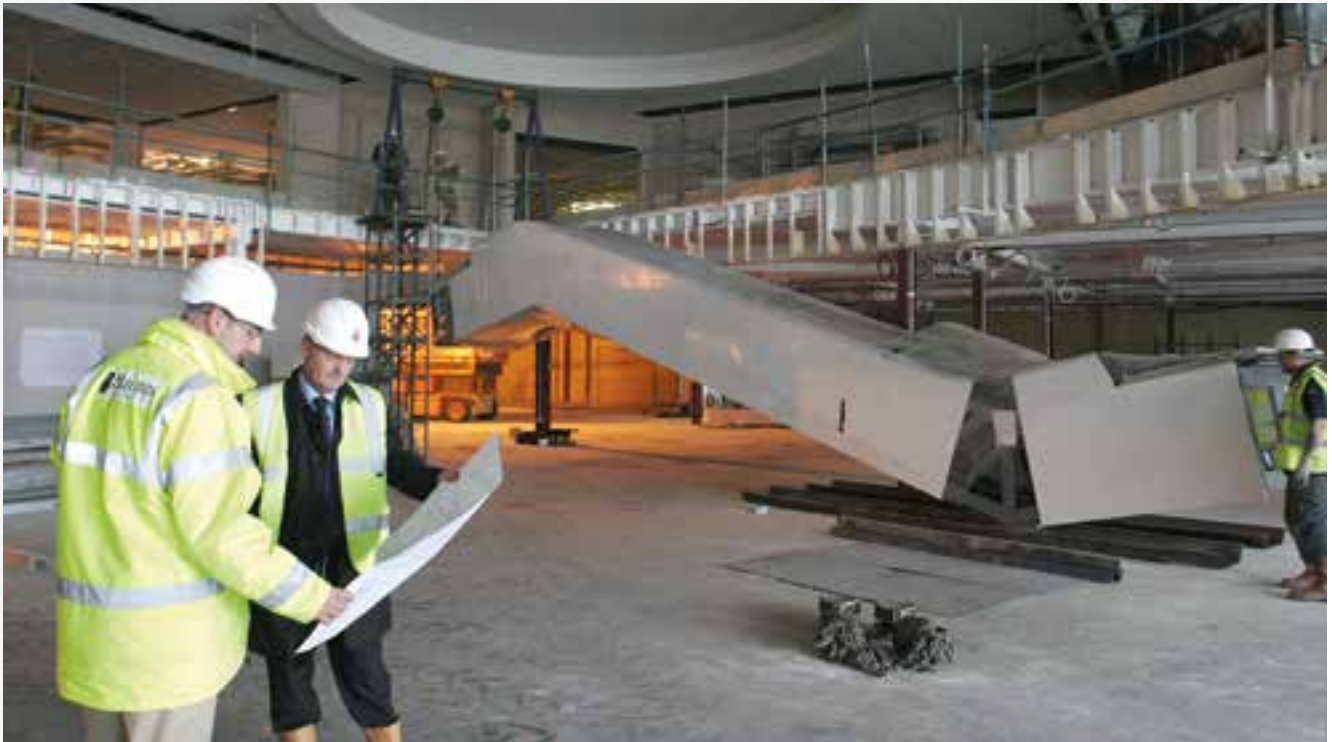
Installation of the escalator.
