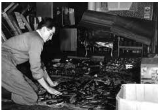
Mending the floor in the Corn Exchange Showroom.
