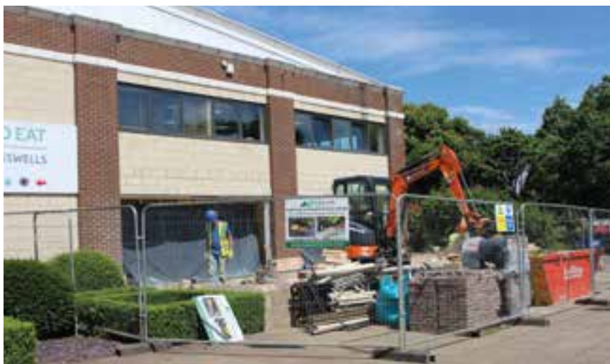
Building of the restaurant extension at Bury in 2016.
