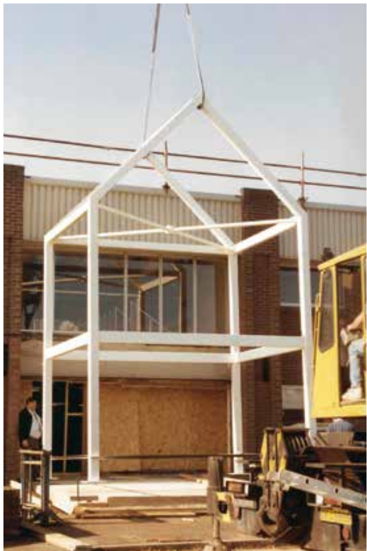
Construction of the new customer entrance.
